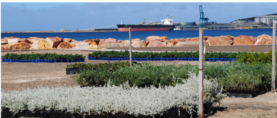
Plants arriving on site in preparation for planting
