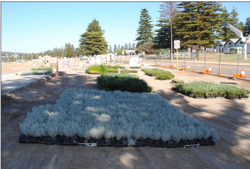
Plant arrival on site in preparation for planting.
