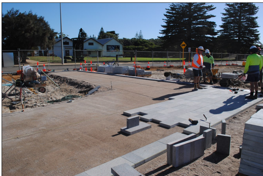
Paving commencing at James Street Plaza
